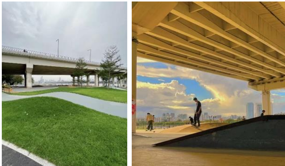
Figure 9: Pazhou Bridge in Guangzhou
