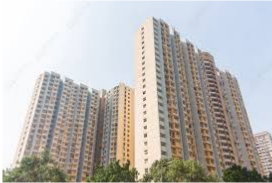
Figure 2. After the renovation of Wong Tai Sin Ha Tsuen
