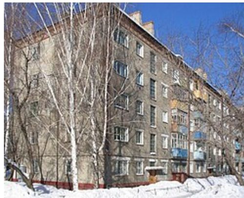
Figure 3. Before dismantling Khrushchyovka
