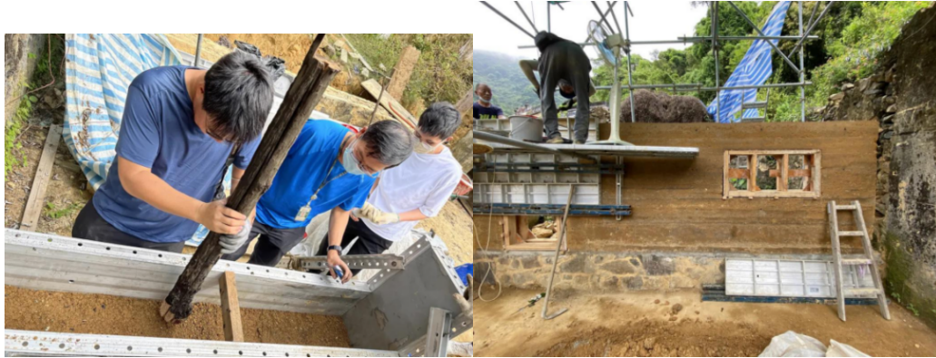
Figure 1. Reconstruction of rammed earth wall
