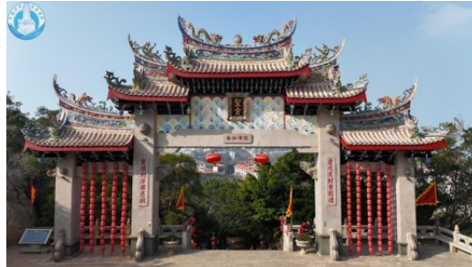
Figure 1: The Shengzhi Gate and Yimen Square
